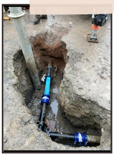
4" Water main replacement on Short Street - March 1, 2024
