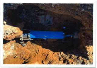
• There is an electrical issue at Harvey tank site. It is in the middle of getting resolved. James tracked it down to water in the conduit boxes located in the tank vault.
