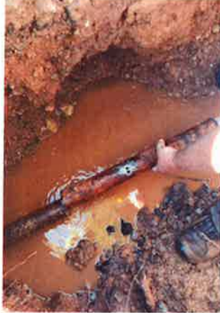
Before 2" main repair.
