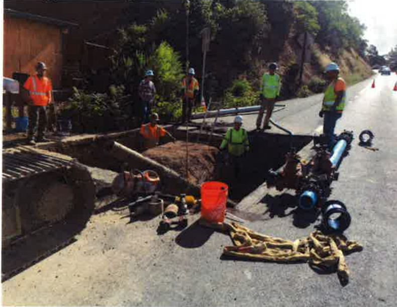
DMA bypass on Hwy 20 and Lakeview Dr.
