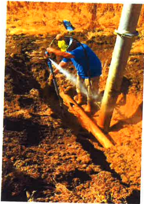
Elem water main before
