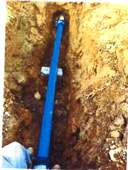
Elem water main after
