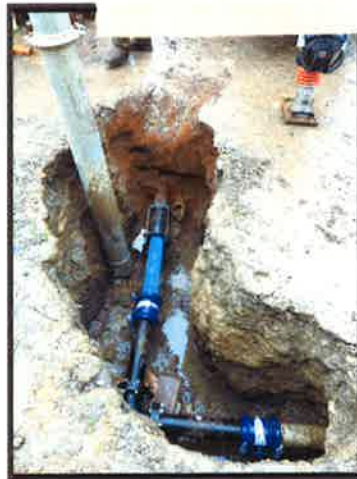
4" Water main replacement on Short Street - March 1, 2024
